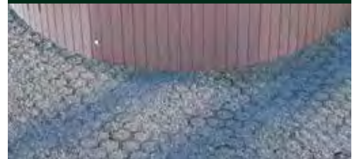
Hot Tub Footing
